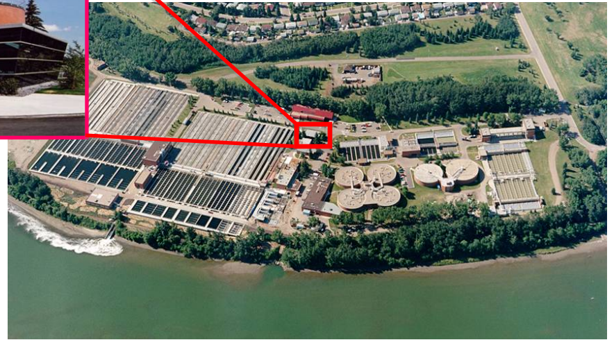
Gold Bar Wastewater Treatment Plant
